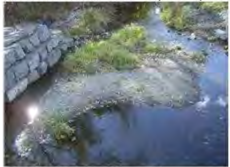
20091031 Stonedust pathway washing downstream at Old Colony Culvert
