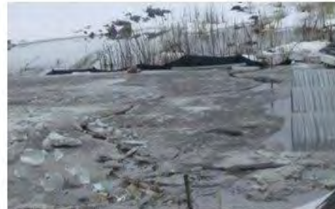
11 Mar 2011 Carp River Culverts at Hazeldean Road
