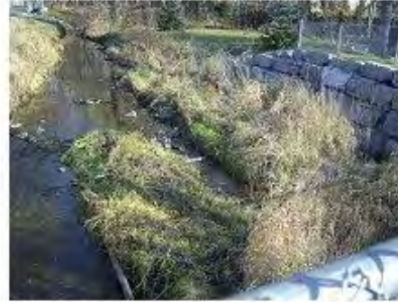
20101119 Sediment build-up since 20 June 2007
