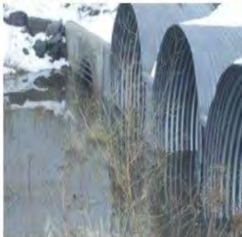
20110311 Terry Fox Culverts
