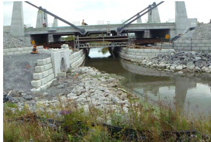
Carp River Bridge 20110930
