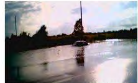
24 July 2009 Terry Fox Drive at Trans Canada Trail - Pond backup and blocked culvert caused flooding
