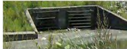
20090814 Castlefrank Twin Sewer outlets in Glen Cairn Pond
