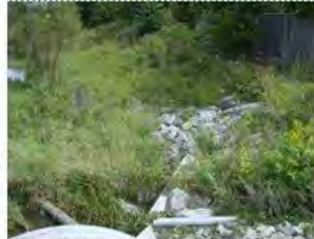
20090828 McElroy Outfall constructed in 2002/3
