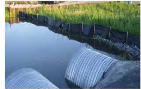
25 June 2010 Carp River culverts at Hazeldean
