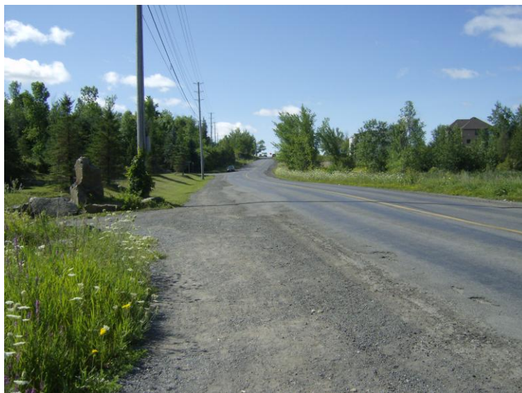
GFR Hill to the north with sloped road shoulders
