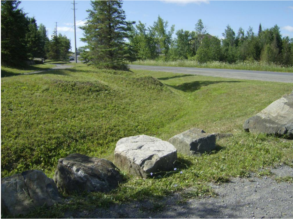
GFR east side ditch adjacent to The Rockeries. Flow is coming down the ditch system from the top of the south GFR hill
