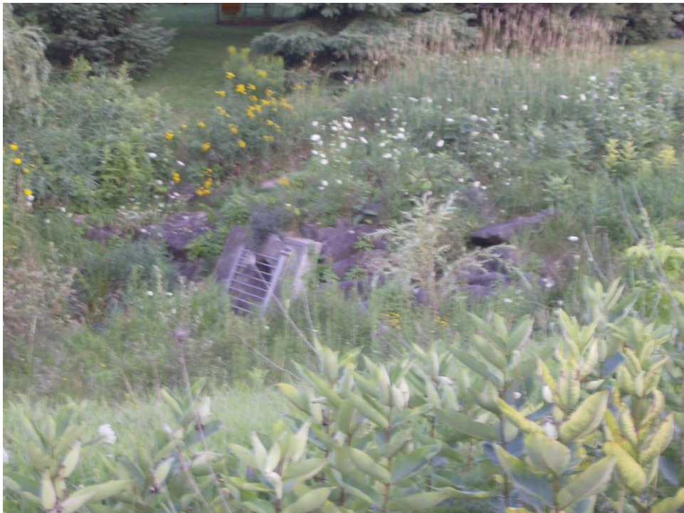
This is Beaver Pond outlet in the north Watts Creek channel
