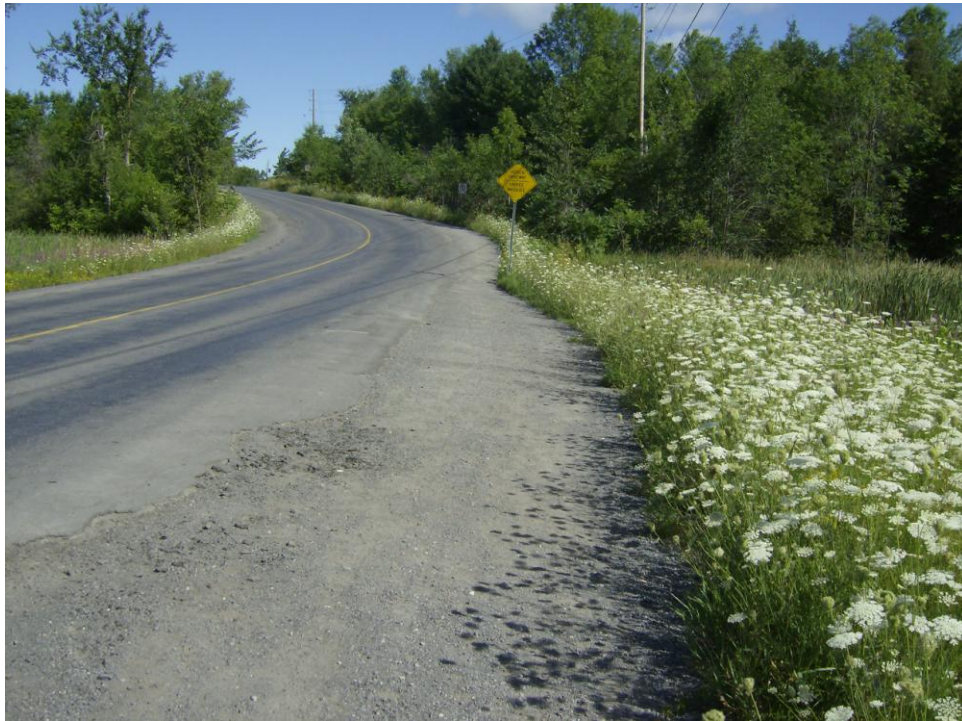
GFR hill to the north; sloped road shoulders drain to Beaver Pond
