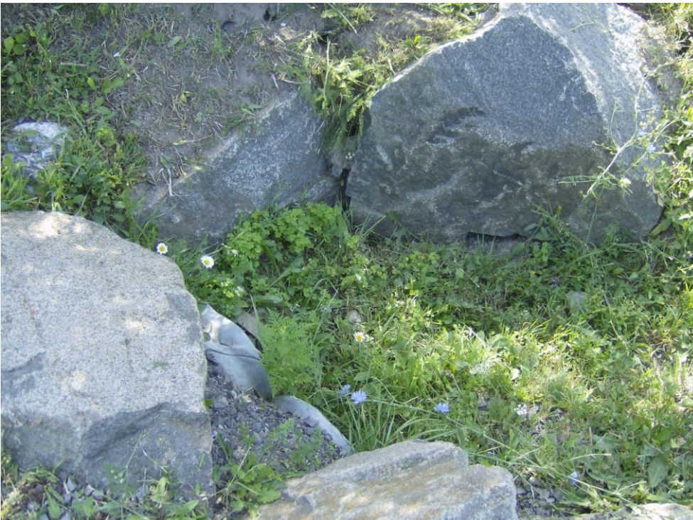
Twin CSP culverts at the pathway receive stormwater from the east side GFR ditch. Ponding would occur here in extreme events.
