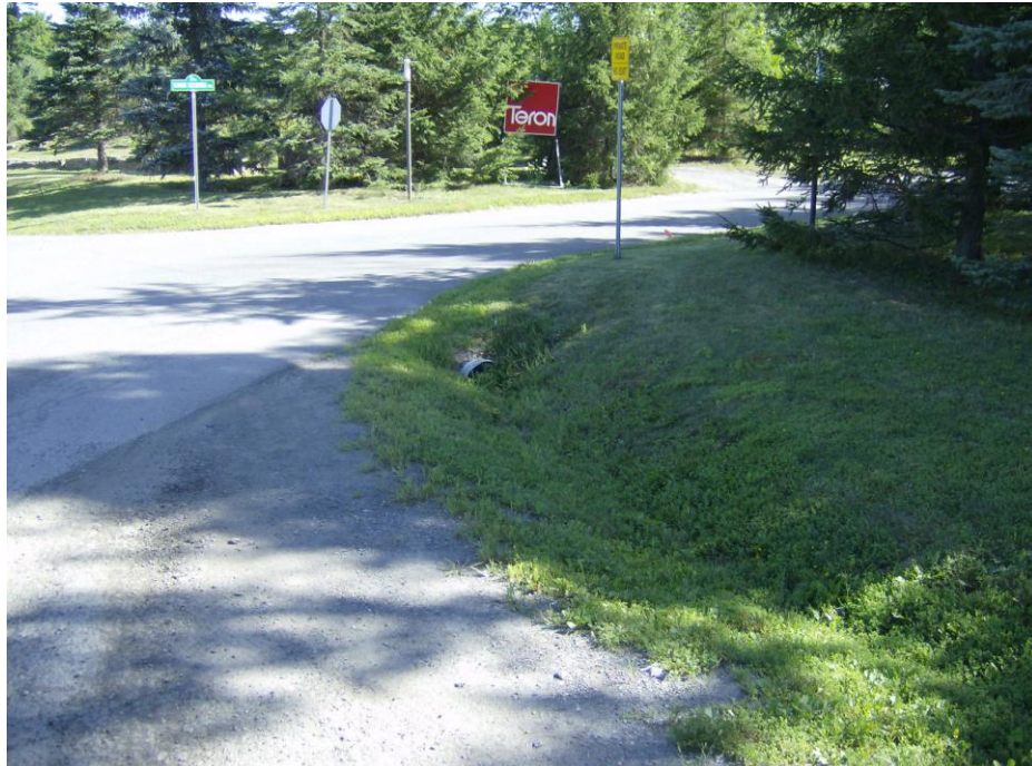
Culvert in GFR east-side ditch goes under the private road
