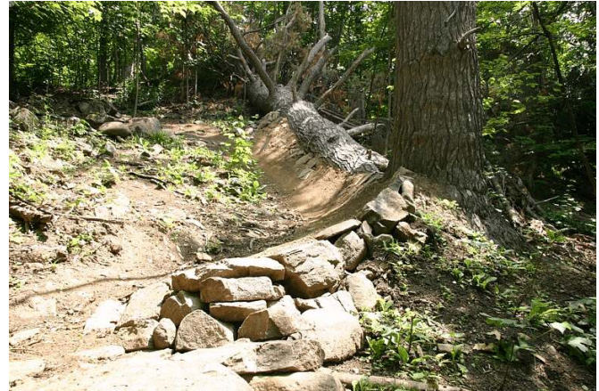
Figure 30: chute constructed along trail near Huntmar Road for mountain bike racing
