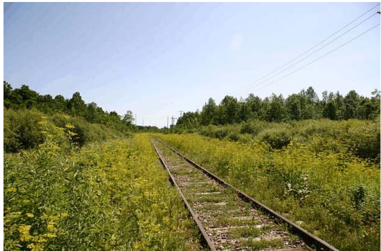
Figure 23: railway corridor eastward from First Line Road ROW
