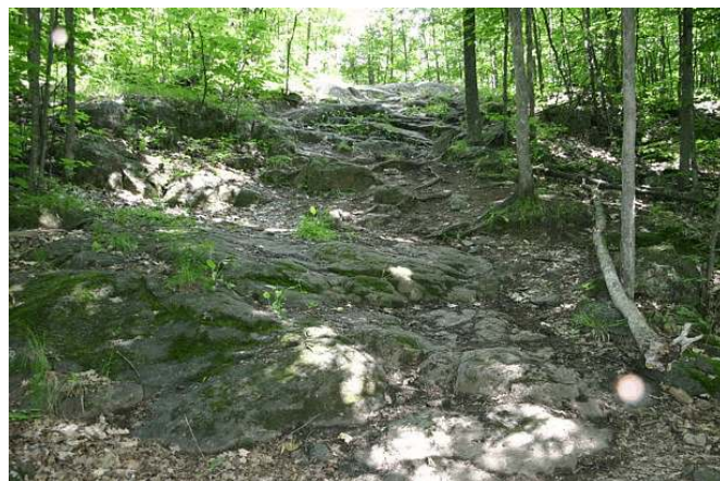
Figure 25: severe slope erosion to bedrock along mountain bike trail
